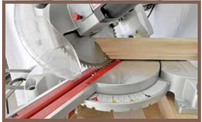
Miter cut the decorative moldings at 45-degree angles where the face section joins the return section. Remember to use the outside measurement of the face board for the inside cut of the miter.
